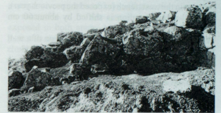
Fig. 12: North facade of stonewall M13.
